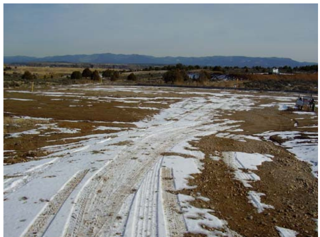
Access at Road
