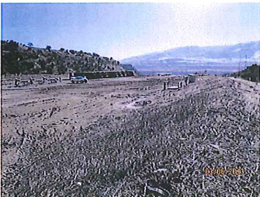
PAD OVERALL LOOKING SOUTHERLY
