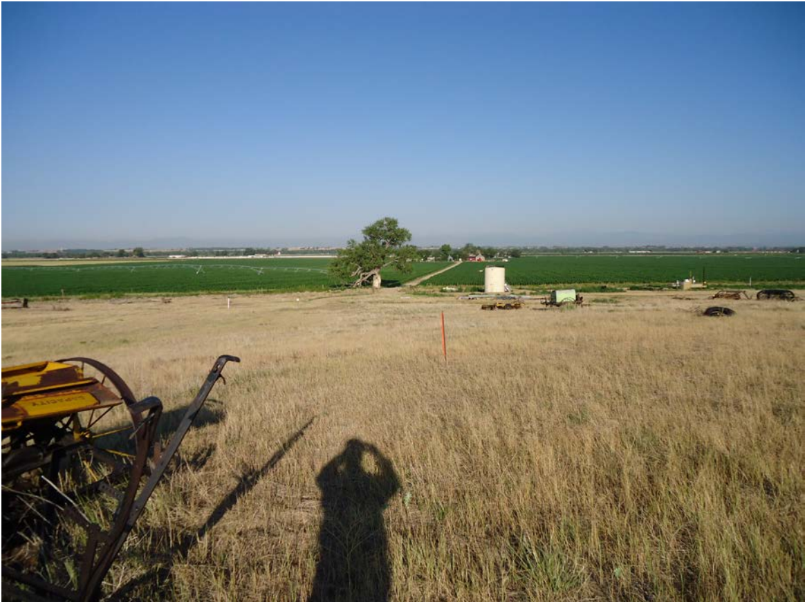
KUNZMAN FEDERAL TANK BATTERY 35N-8HZ
