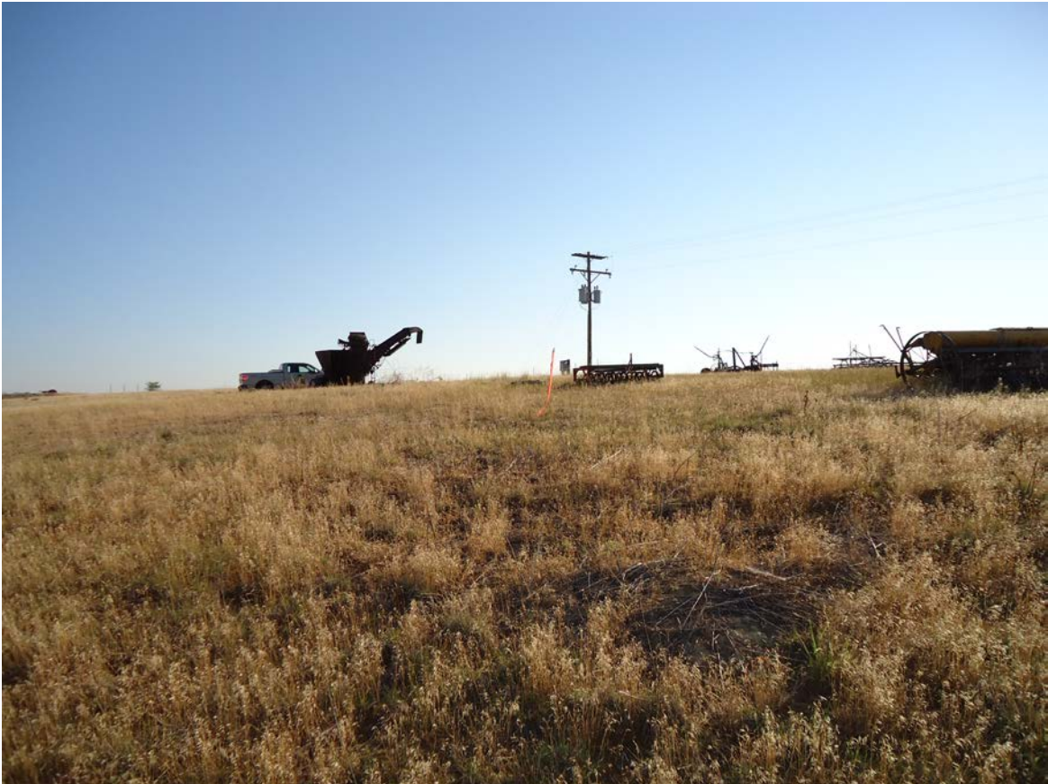
KUNZMAN FEDERAL TANK BATTERY 35N-8HZ
