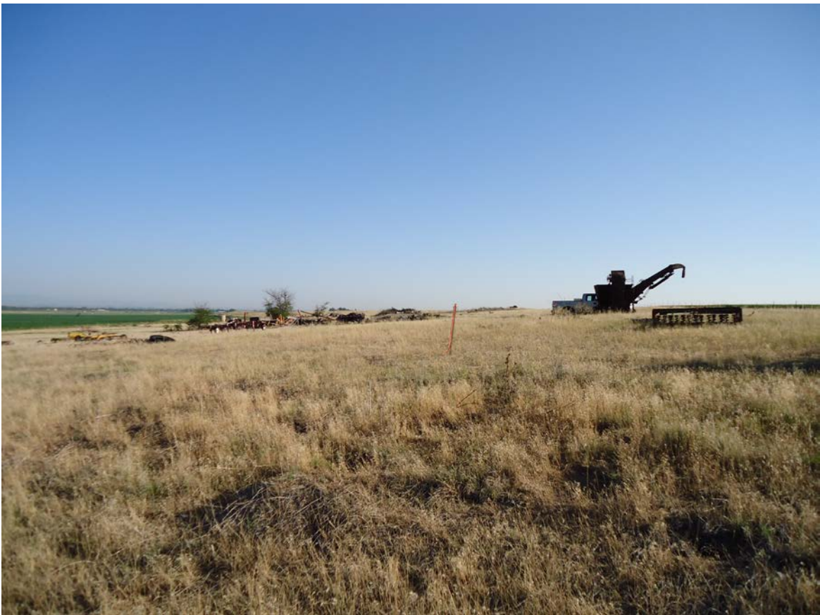
KUNZMAN FEDERAL TANK BATTERY 35N-8HZ SESW Section 5-2N-66W
