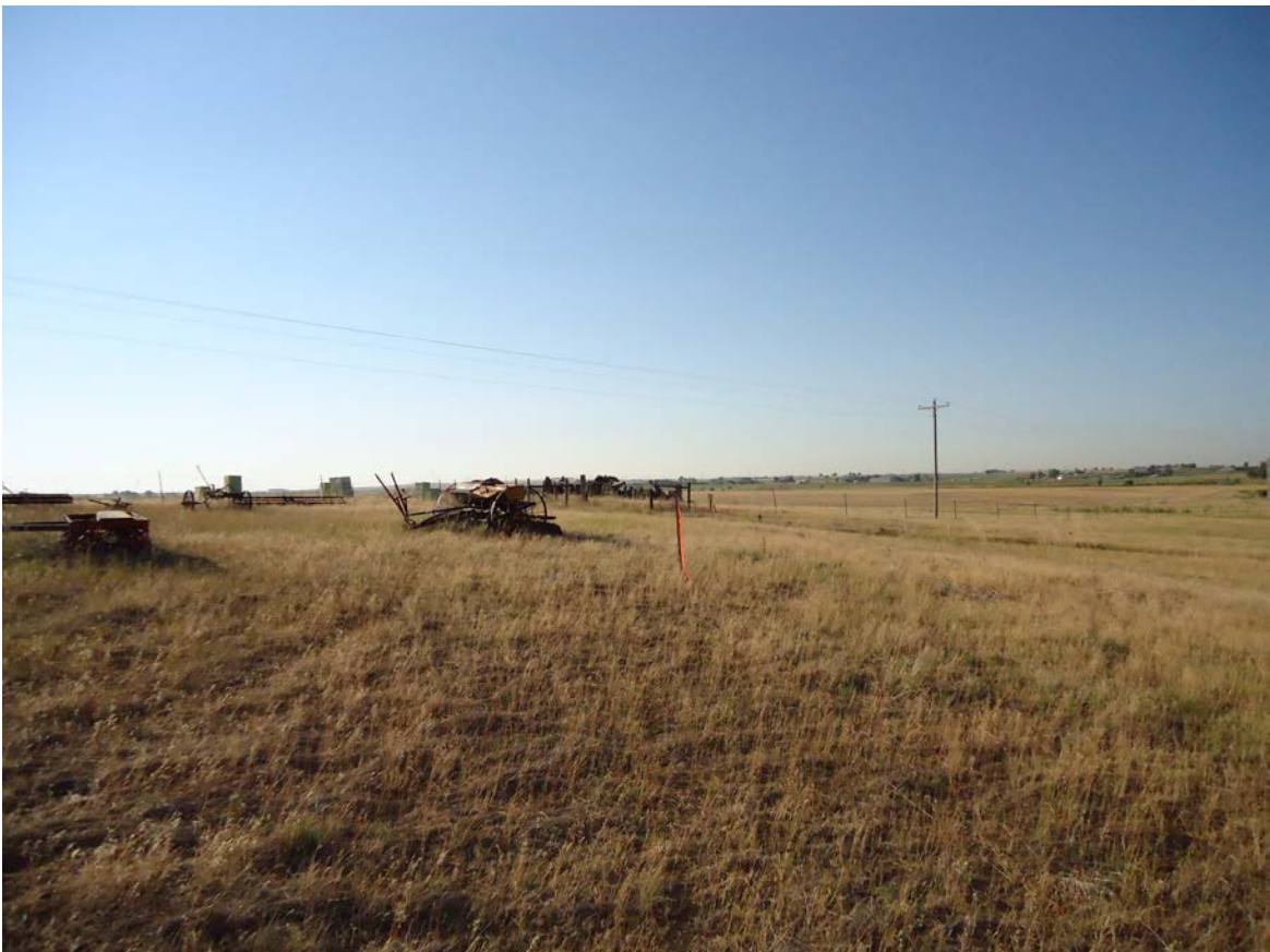
KUNZMAN FEDERAL TANK BATTERY 35N-8HZ
