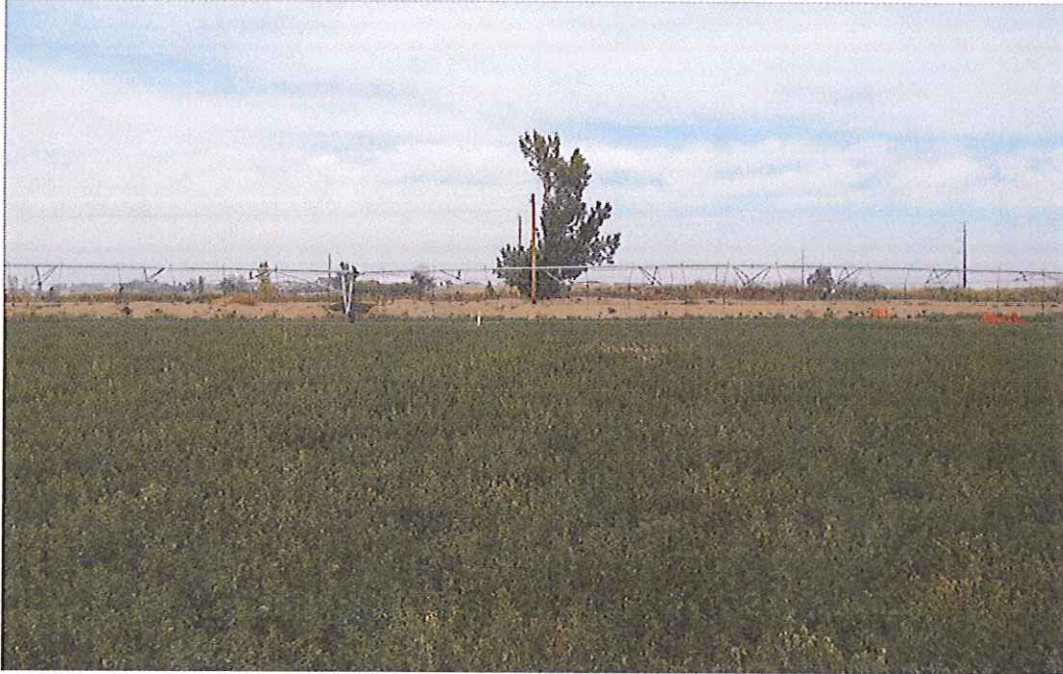
PHOTO: VIEW OF OFFSITE TANK BATTERY
