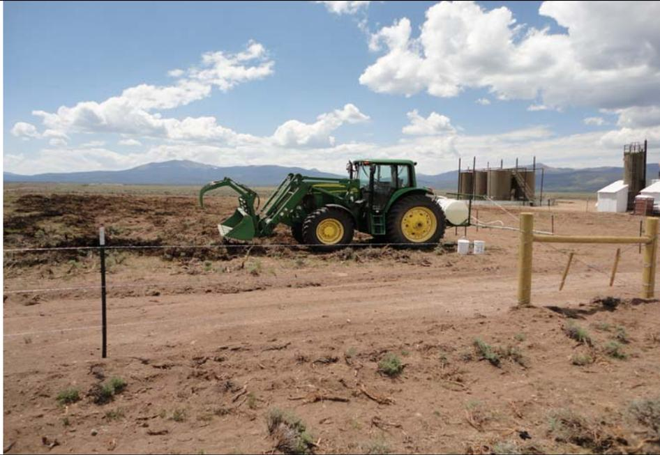
**Subject:** A John Deere 741 tractor with a 150-gallon capacity polytank and a sprayer boom was used to apply the EarthSmart hydrocarbon cleaner over the impacted area. The vertical separator is shown at the right hand side of the photo. A three-strand wire fence had been constructed to keep cattle out of the area.
