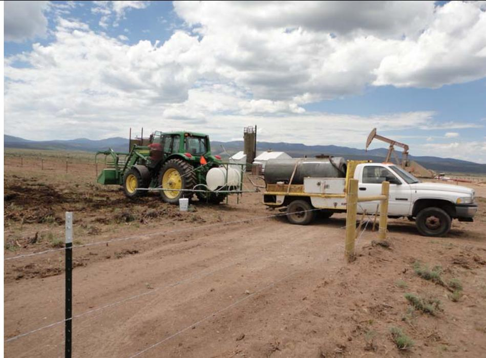
**Subject:** Water was obtained from a pond on the Fuqua Ranch and brought to the site in a 1,000-gallon capacity tank. The 150-gallon capacity polytank on the tractor was filled using one 5-gallon bucket and approximately 100-gallons of water for each mixture. The area was treated using two applications of the EarthSmart hydrocarbon cleaner solution.
