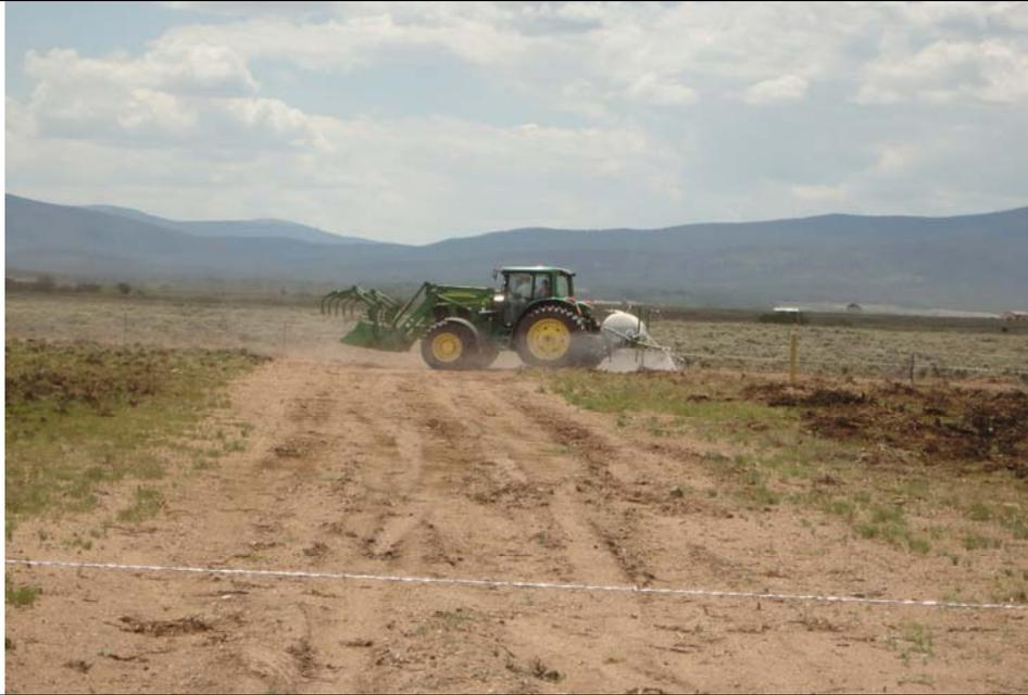
**Subject:** Photograph shows the treatment in progress near the stockpile on the south side of the release area. A fire break had been cleared around the release area since the original treatment plan was to burn the impacted vegetation. However, Jackson County implemented a fire ban due to a lack of precipitation and high fire danger.
