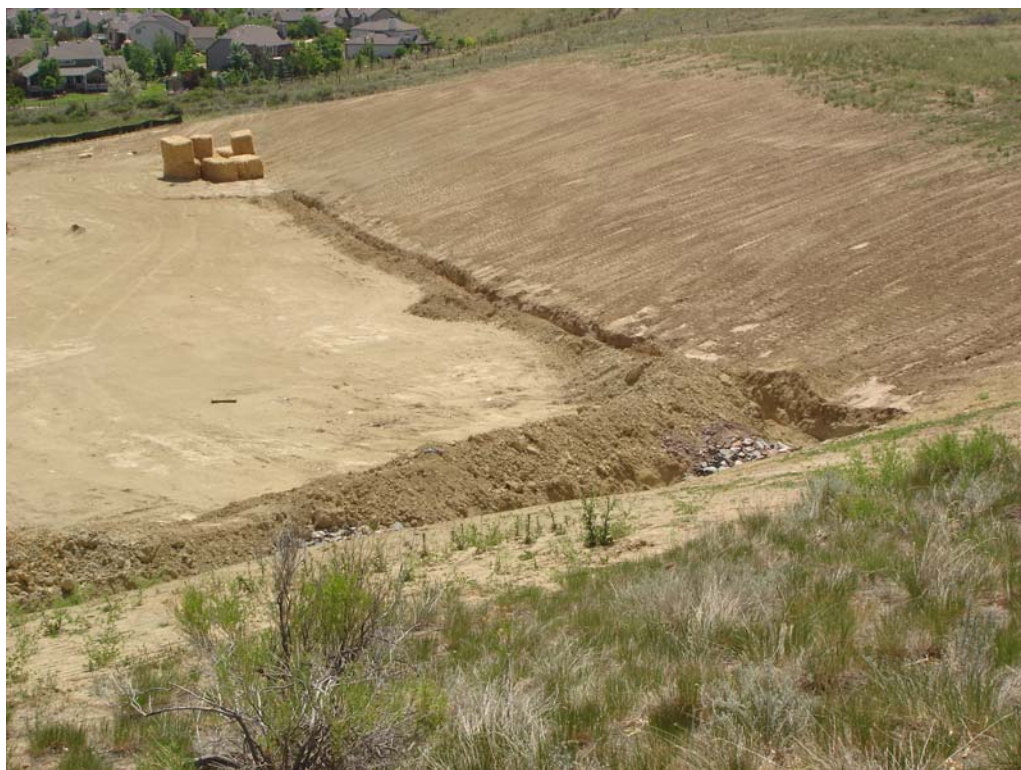
5/30/12 Photo of discharge for “run-on” control ditches
