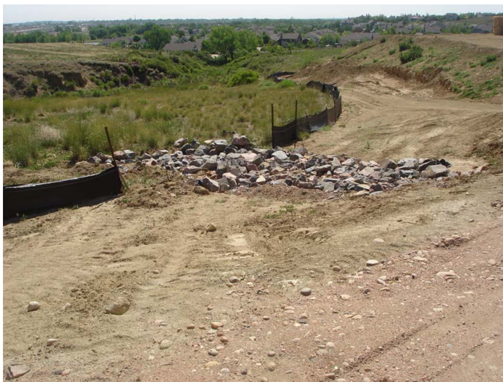
5/30/12 Photo of discharge for “run-on” control ditches
