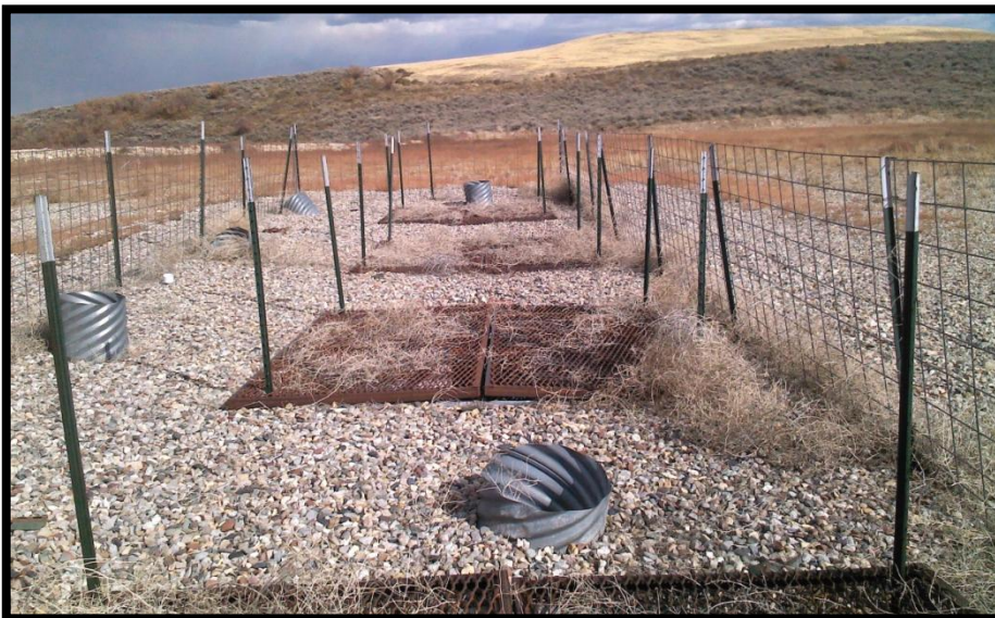
Viewing East: ratholes & conductors (capped & w/grates over cellars
