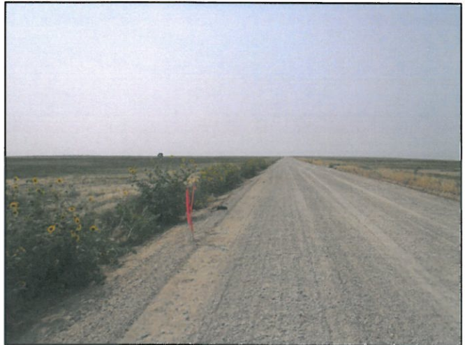
Looking down the roadway to the left of the access
