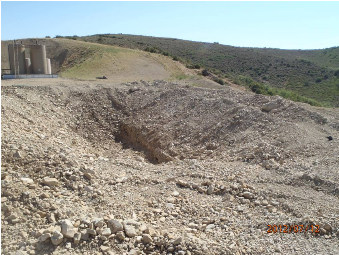
Visual representation of the impacted soils on pit bottom and pit walls post excavation
