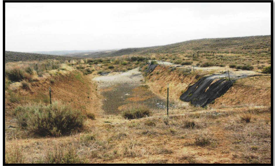
Viewing Southeast: drill pit, lining & fencing conditions
