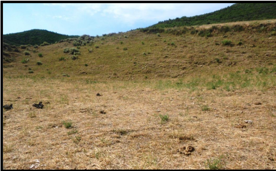
Viewing South: well pad footprint, with partial vegetation, and cut slope, and surface modification to promote revegetation.
