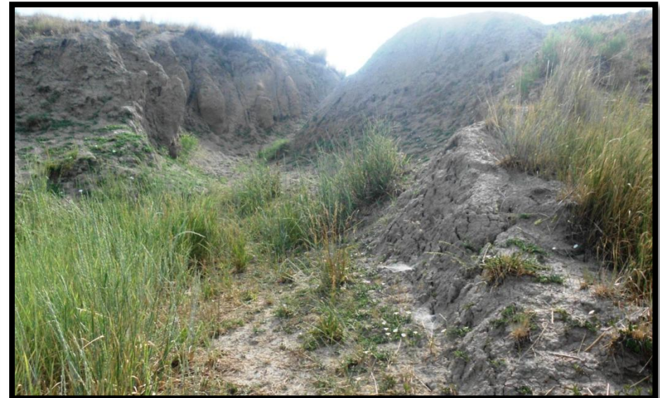
Viewing east: Large Gully wash that originated from top of fill slope.
