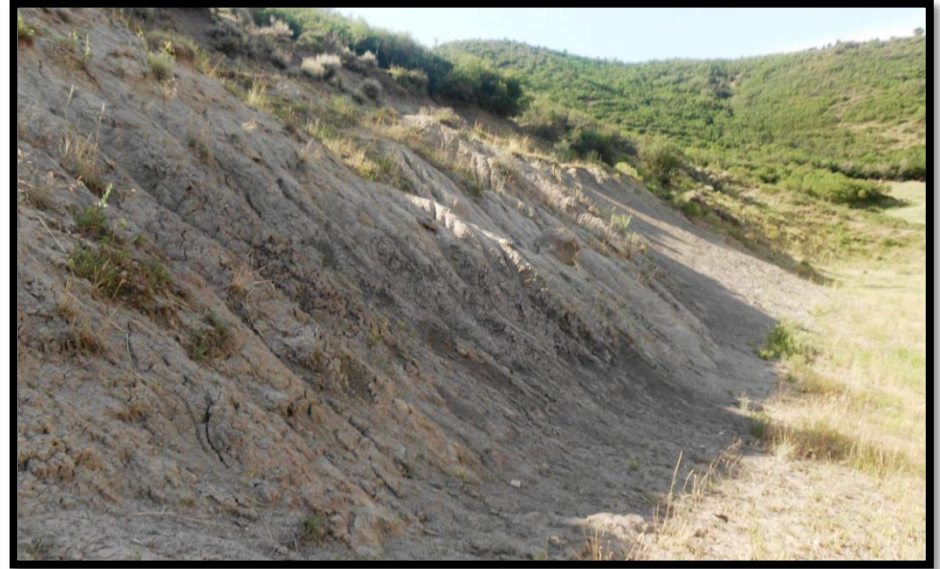
Viewing southeast: Rill formation along cut slope.
