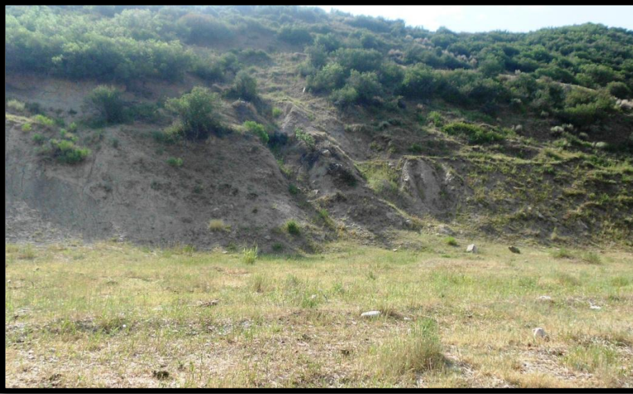
Viewing east: Gully erosion along cut slope.
