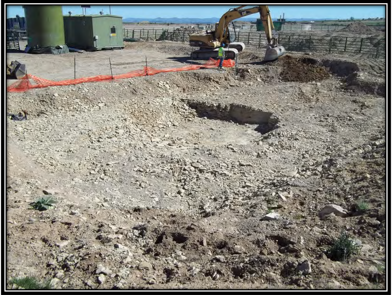
PCU 296-7A Former Tank Containment Area – Following Initial Soil Removal
