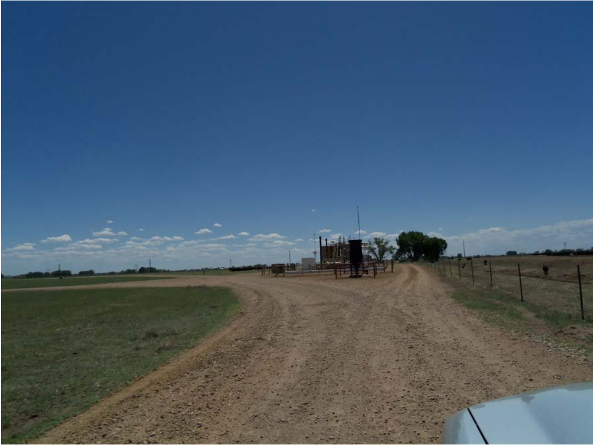
CANNON TANK BATTERY 36N-W3HZ
