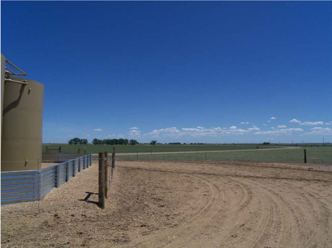
CANNON TANK BATTERY 36N-W3HZ
