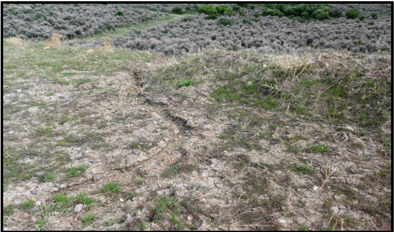
Viewing South near edge of well pad and fill slope: Pathway of erosion channel un-barricaded from low spot in perimeter berm.
