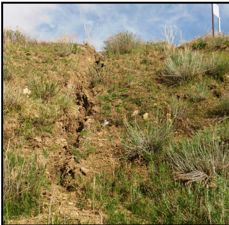
Gully formation on northwest corner of fill slope initiating from top of pad.
