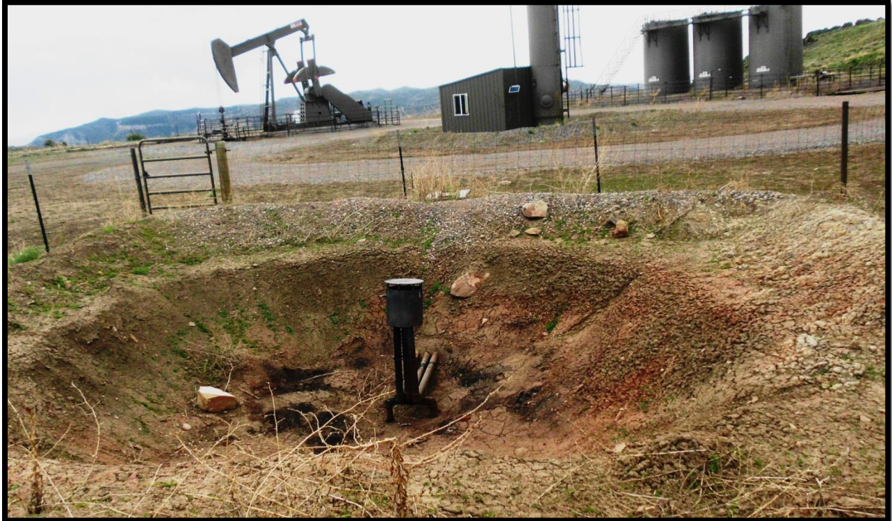
Flare pit: (fenced and bermed).
