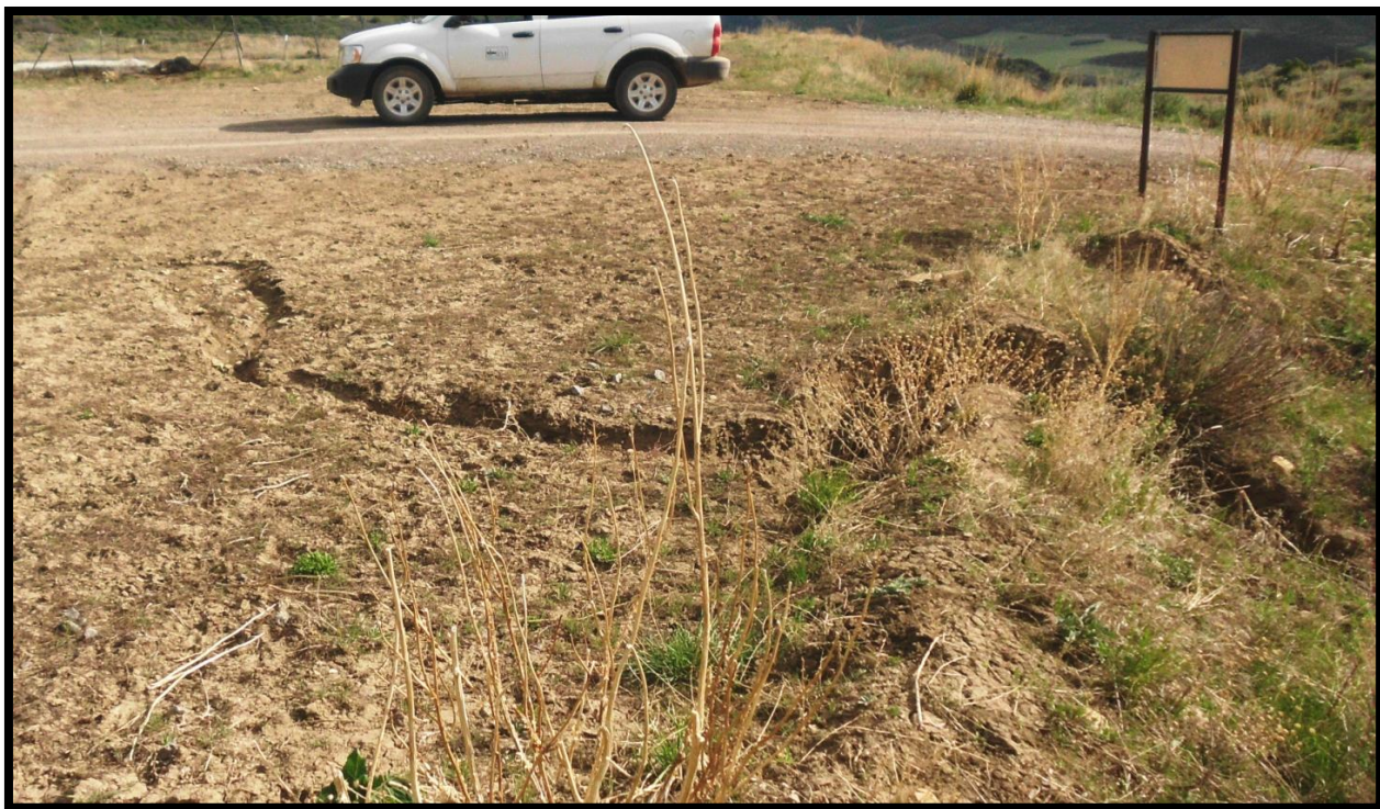
Erosion initiating from northwest corner of pad
