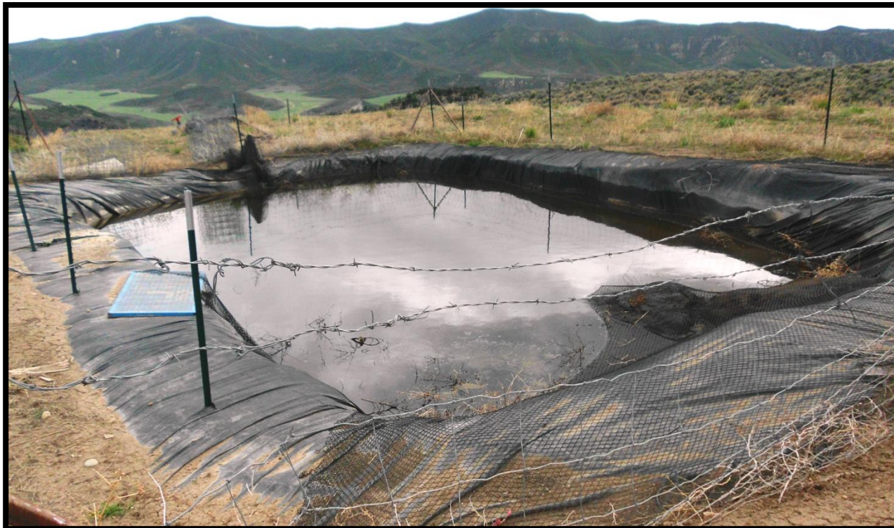
Viewing southwest: "Secondary pit" comprising of produced water with condensate. Approx. 25' x 40'.
