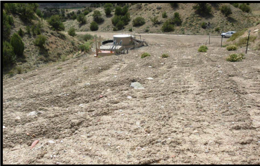
Disturbed surfaces to the east has no vegetation or erosion control BMPs .
