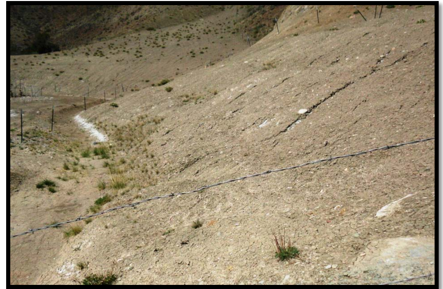
Viewing north: Cut and side slopes experiencing rilling. Negligible vegetation observed.
