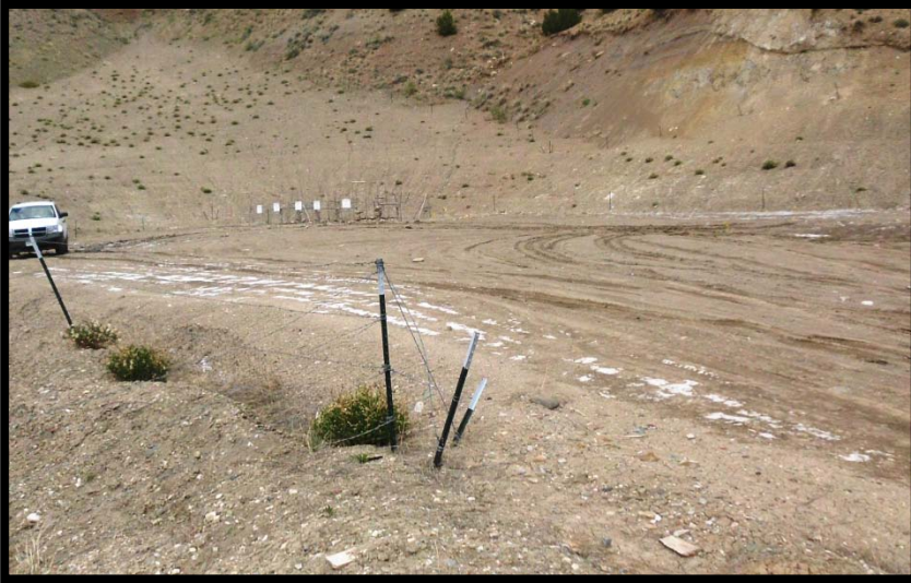
Viewing north: Cut slope experiencing rilling. Negligible vegetation observed.
