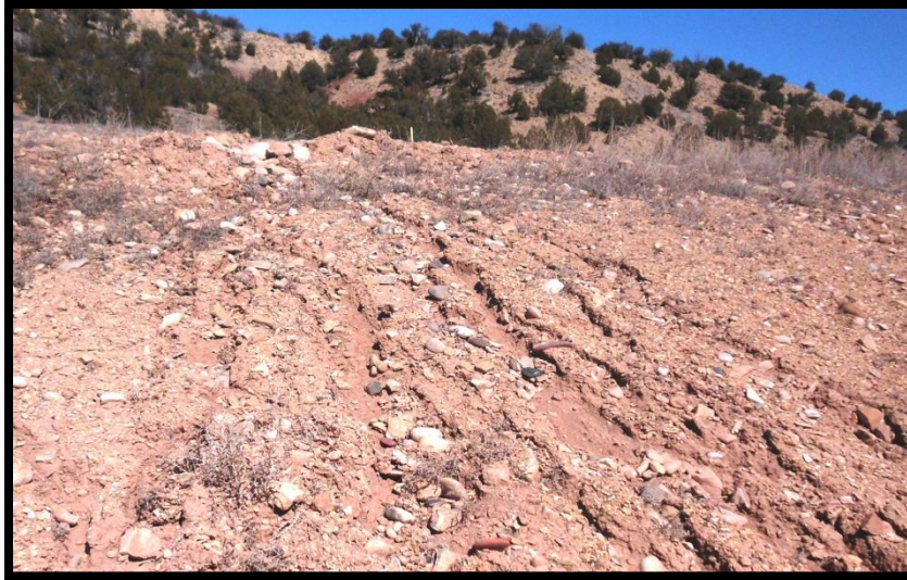
Viewing northerly: Rill erosion along fill slope
