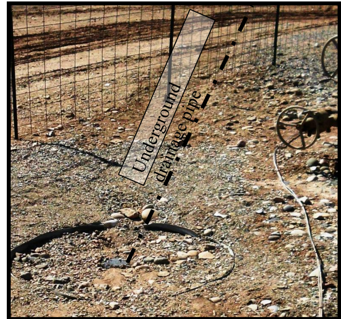
Viewing northerly: pipe outlet & riprap on fill slope
