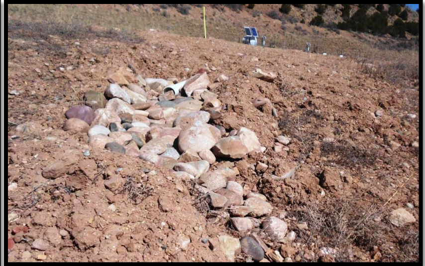
Viewing northerly: pipe outlet & riprap on fill slope
