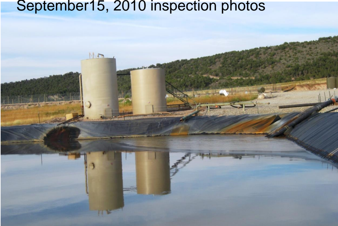
Viewing North: Williams Jolley Pit 301014: Tanks have negligible gravel berms. Further north is the BBC Jolley #1 Pit.
