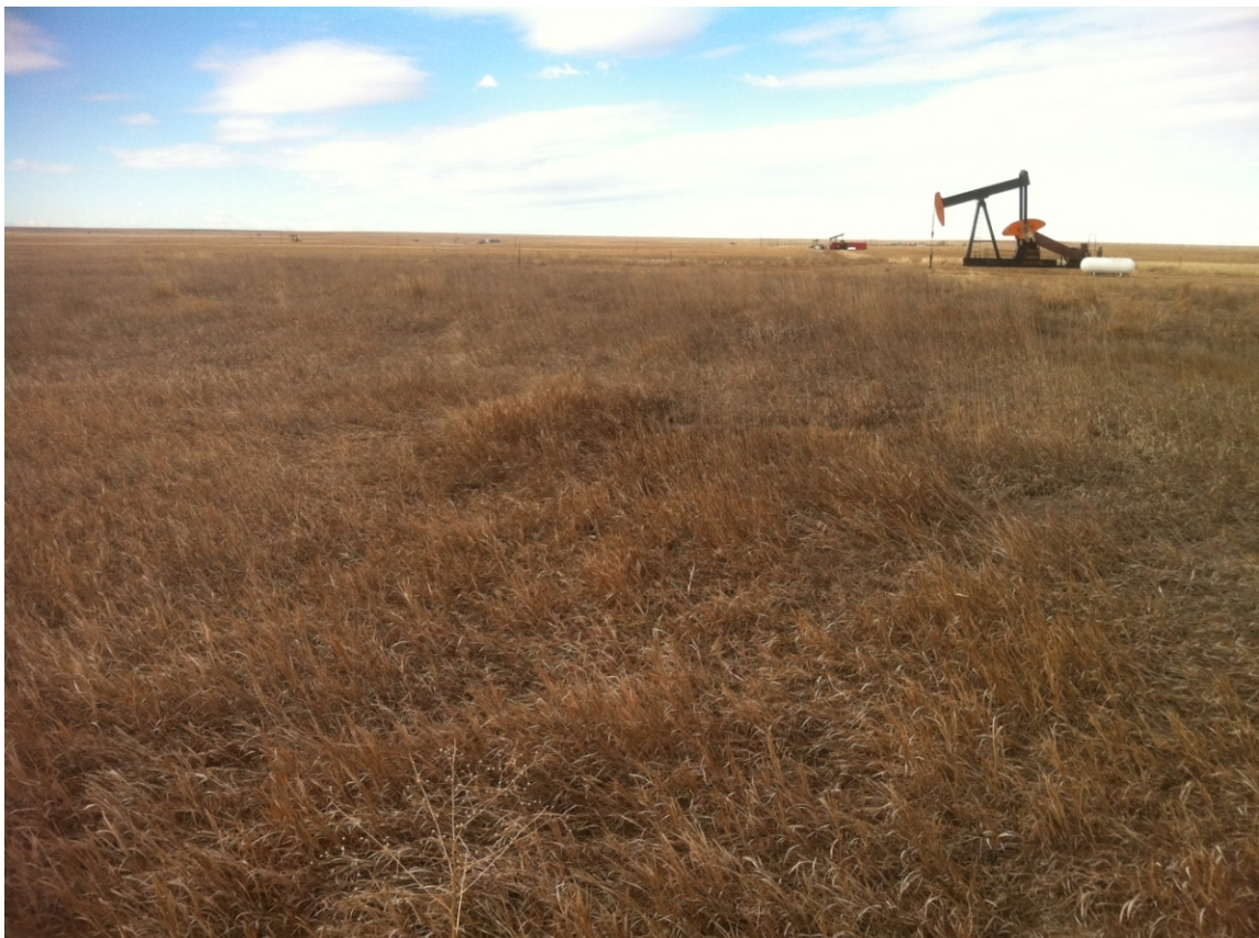
Hough J Sand Tank Battery Location Looking West January 20th, 2012
