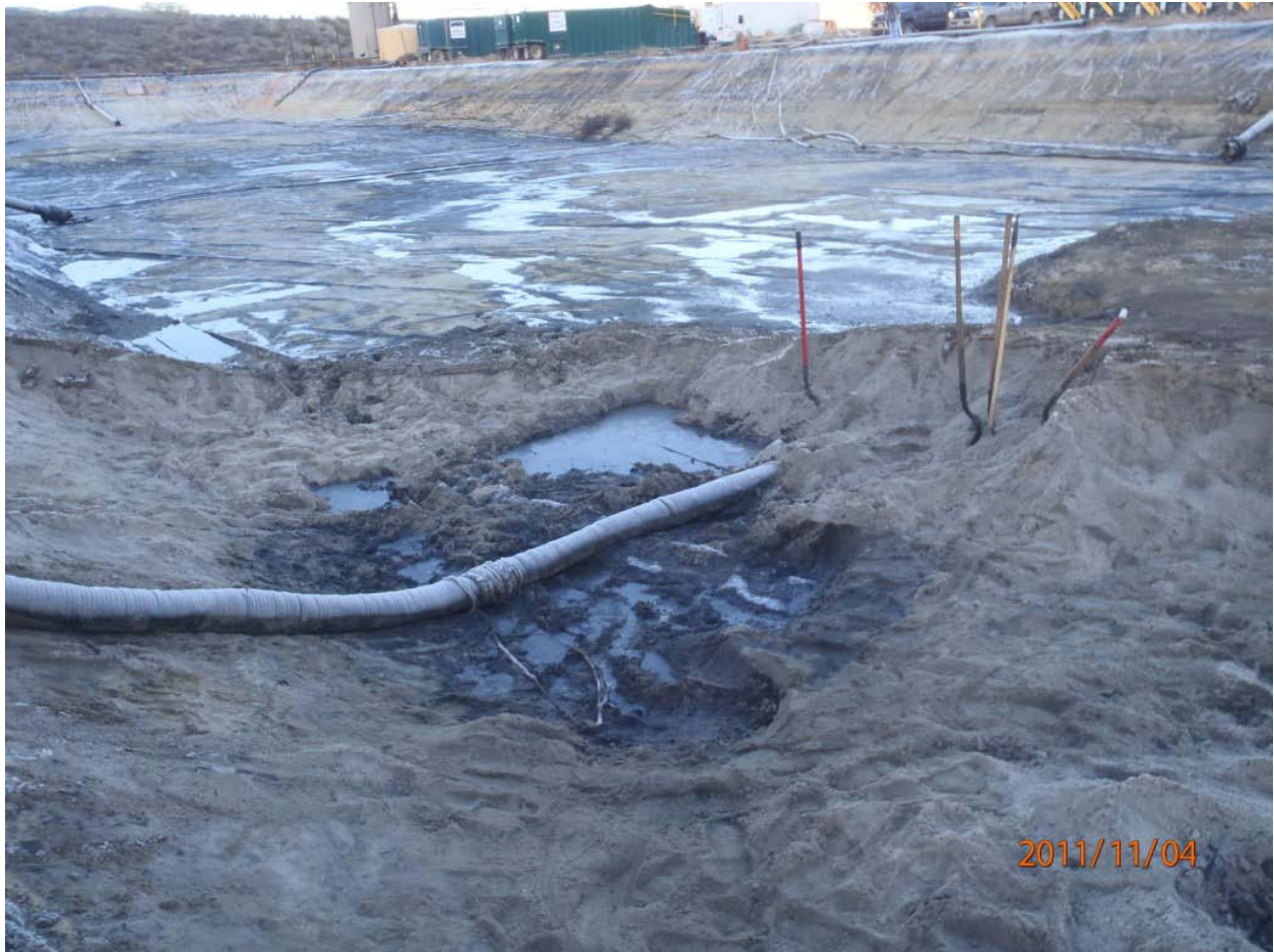
Visual representation of the soil and sand present above the liner in the southeast corner.
