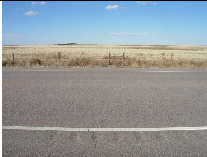
ACCESS OFF HIGHWAY 14
