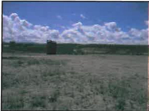
PAD OVERALL (SOUTH)
