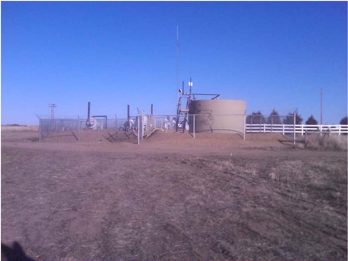
Overlook Tank Battery 27-30
