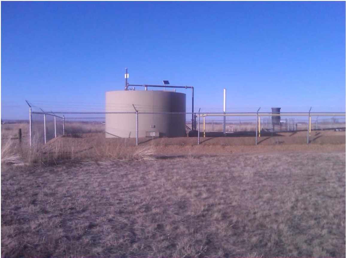
Overlook Tank Battery 27-30 Location North SENE Section 30-2N-67W 02/24/11
