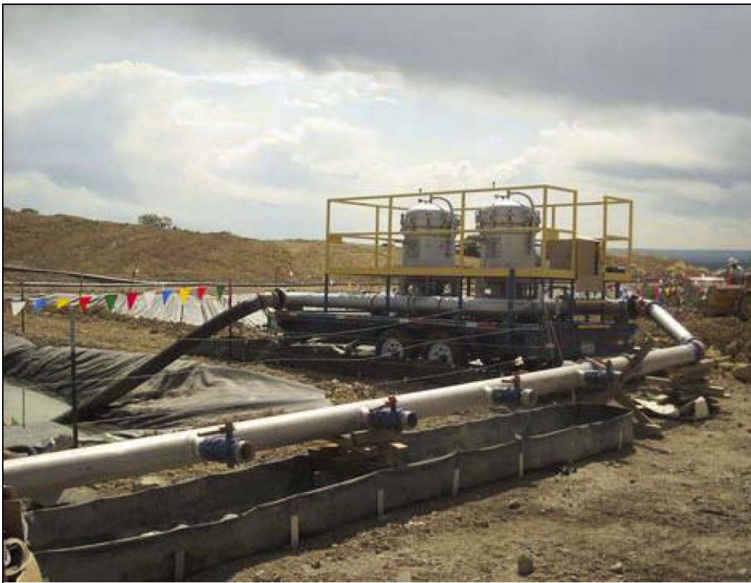
Photo 4. Hose manifold system.
