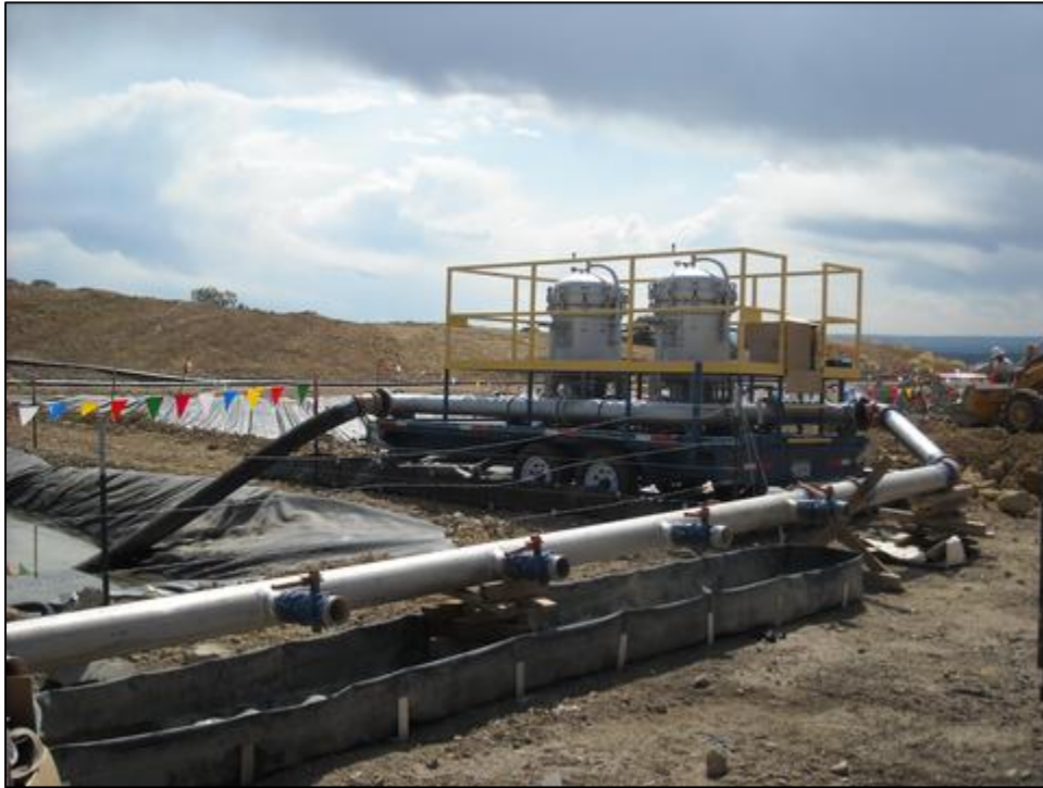
Photo 4. Hose manifold with containment system beneath connections.
