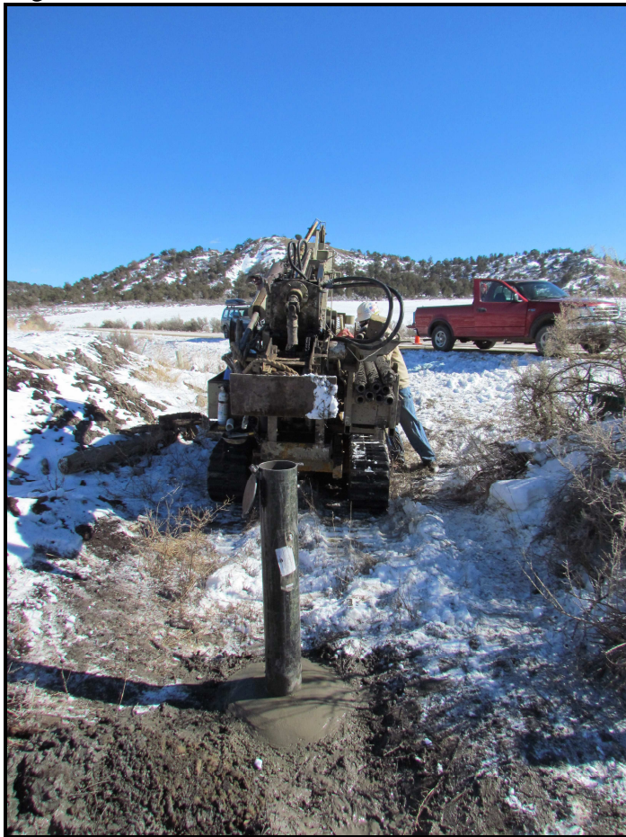
Figure 2. Typical monitor well with steel riser cover cemented into ground.
