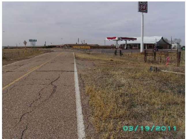
PROPOSED ACCESS FRONTAGE ROAD I-76 LOOKING WEST
