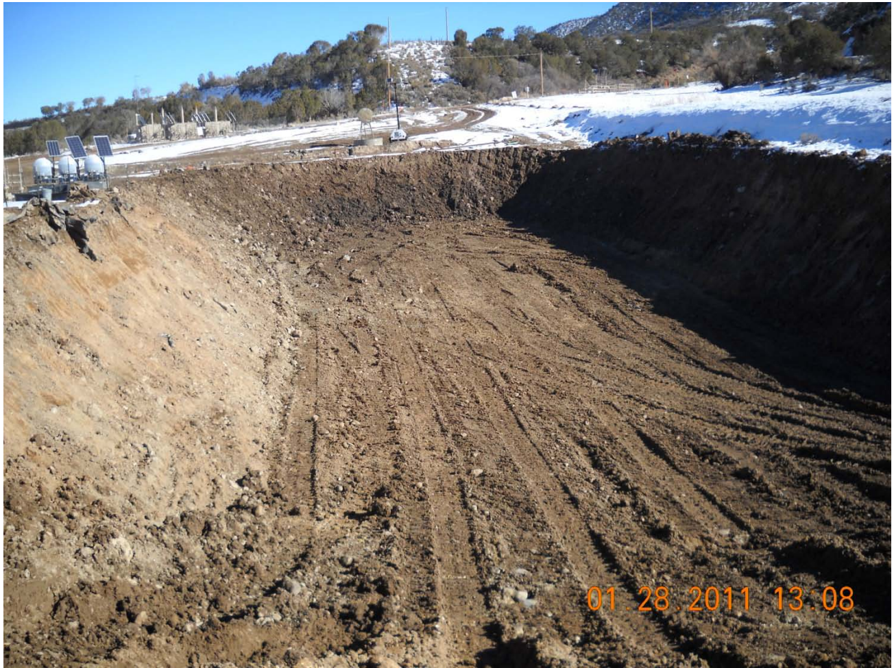
Visual Representation of the Pit Facing East During Excavation
