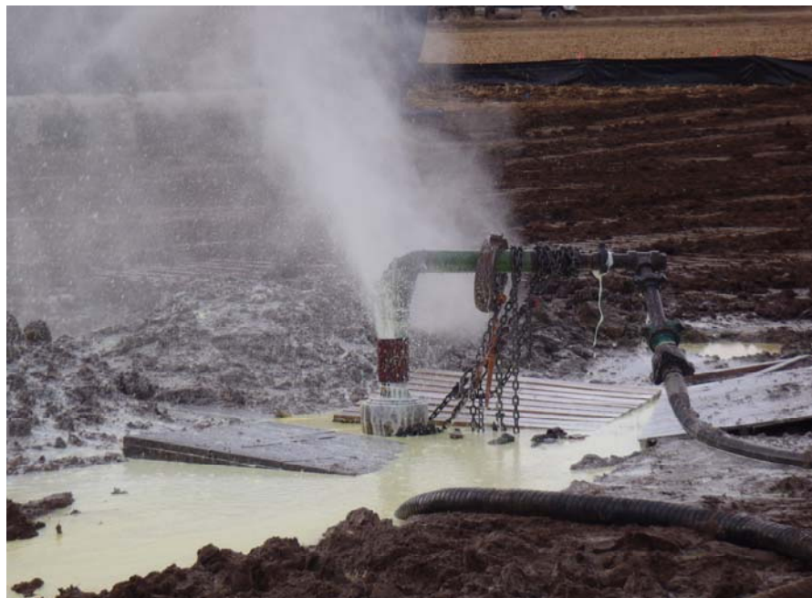
Great Western 25-52 March 2, 2011 – Flow Diverter hooked up to flowback tank
