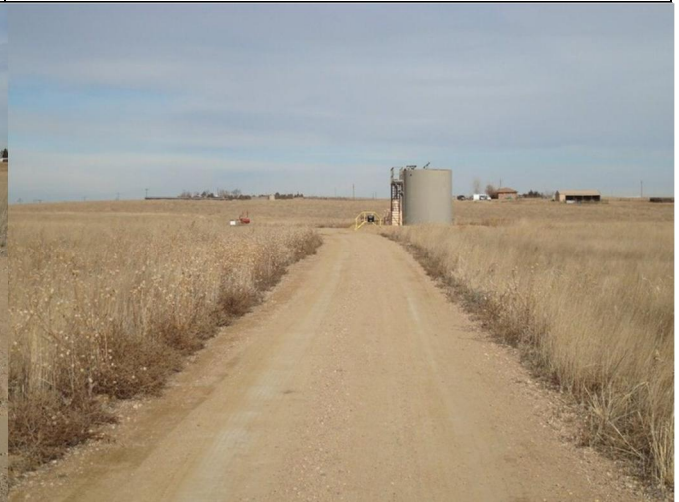
ACCESS TO PAD
