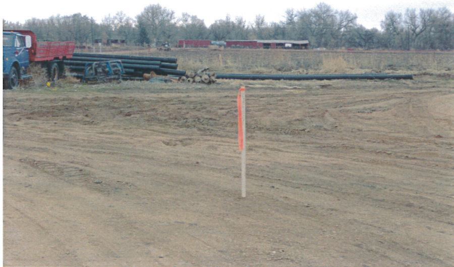
Facility location facing north Picture Dated: 03/08/2010
