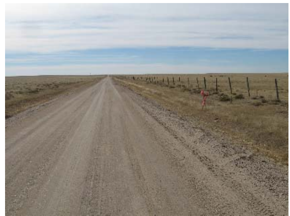
PROPOSED ACCESS COUNTY ROAD 103 LOOKING SOUTH
