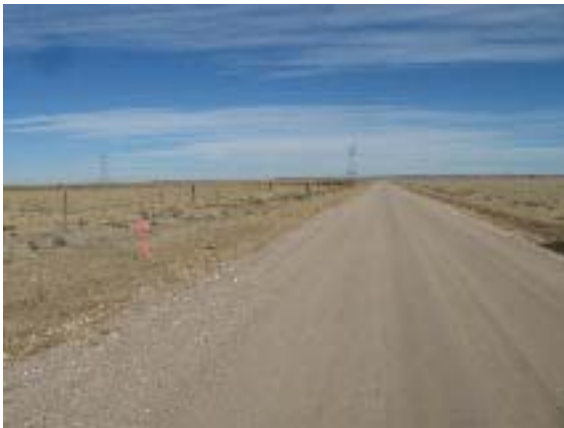
PROPOSED ACCESS AT COUNTY ROAD 103 LOOKING NORTH
