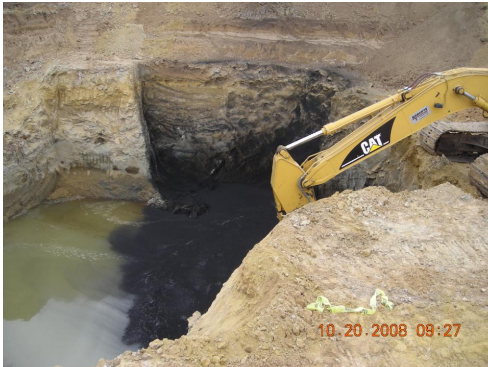
Photograph 3: Installation of hydrocarbon degrading amendment in the northern excavation.
