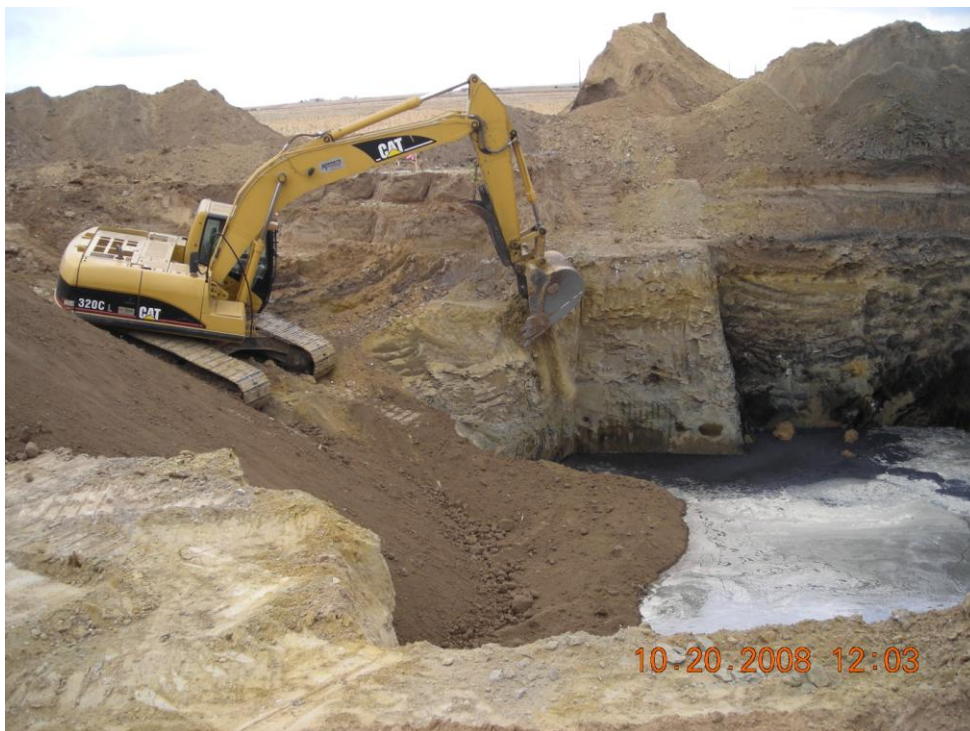
Photograph 4: Backfilling the northern excavation.
