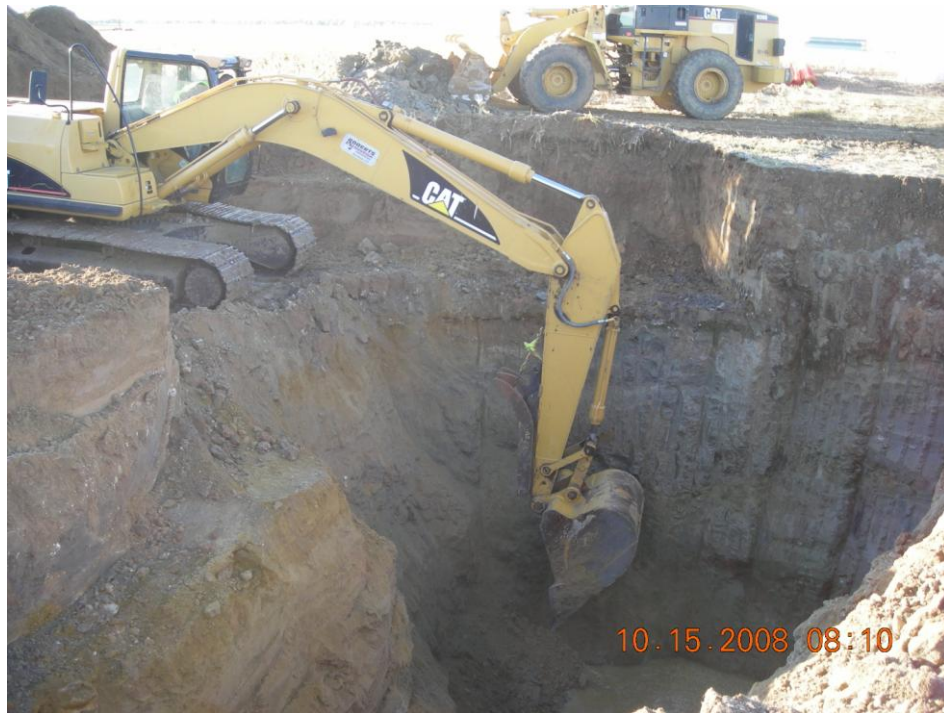
Photograph 1: Excavation of impacted soils at the northern excavation.
