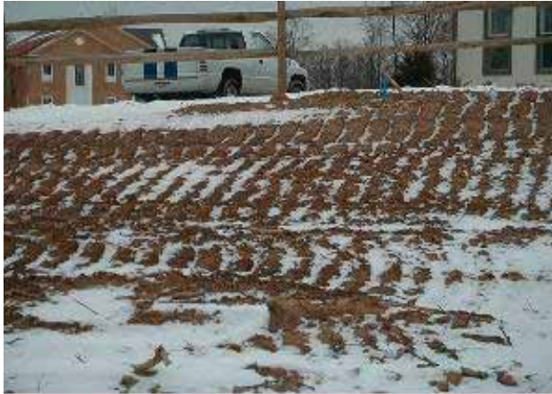
Exposed soils can be temporarily stabilized by driving a tractor over the surface
