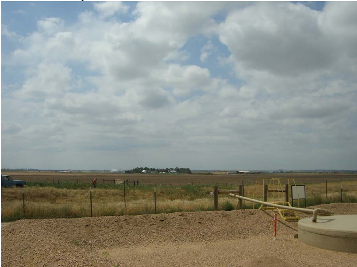
Cannon Tank Battery 24-3
