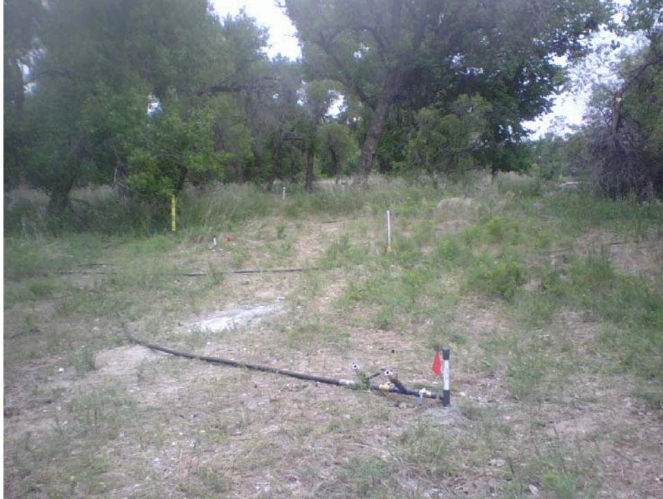
Photo 6: Aboveground air sparging well and associated aboveground piping infrastructure.
