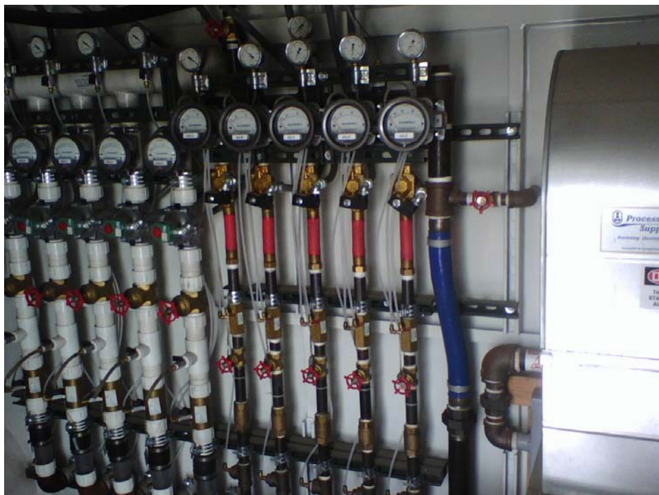
Photo 3: Air sparging/soil vapor extraction manifold. The manifold allows distribution of air in system piping/wells.
