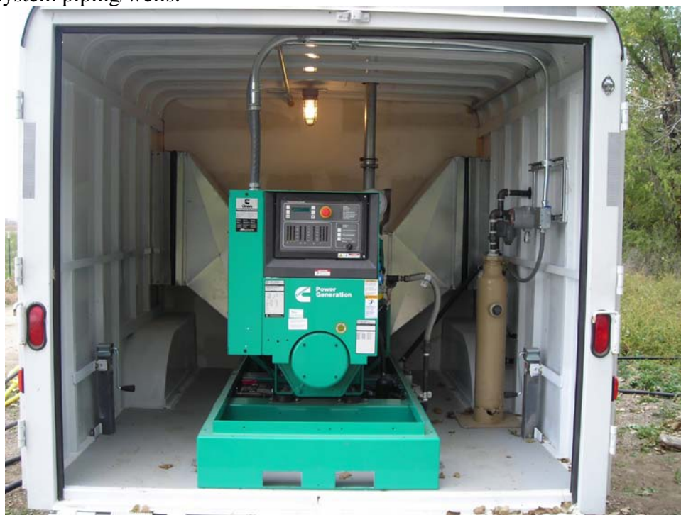
Photo 4: The natural gas generator runs off of wellhead gas, which allows the system to operate in remote locations without electrical infrastructure.
