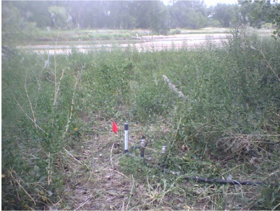
Photo 5: Aboveground air sparging well. The wellhead allows measurement and adjustment of well air flow.
