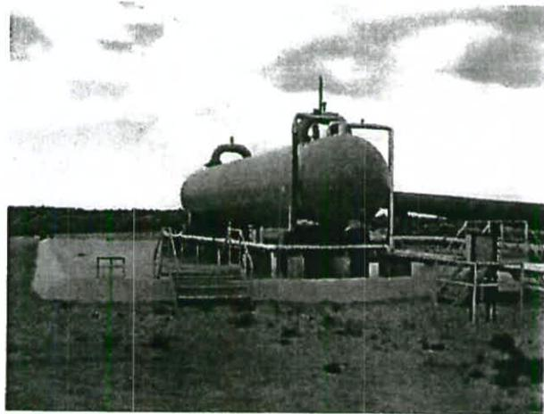
**Custom Linings Containment System takes a durable and easy to place geotextile fabric and combines it with a spray in place, dry in 7 seconds, industrial polyurea containment membrane.**
