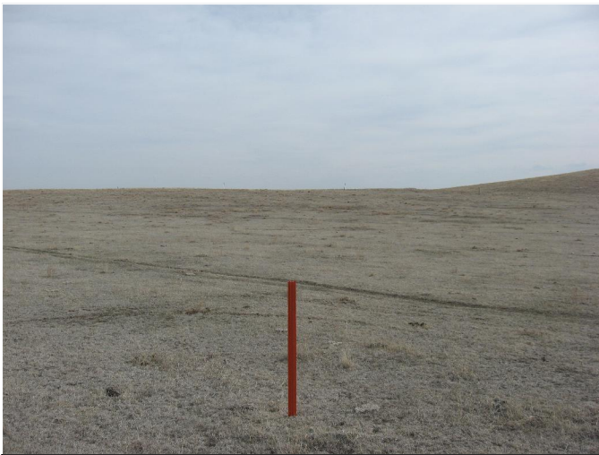
PAD LOCATION FACING SOUTH
