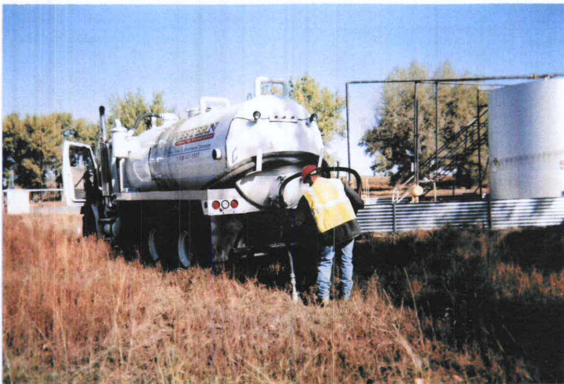
Amen No 1 - Weld County - API # 05-123-10593 Remediating Groundwater via Vacuum Truck Fluid Recovery
