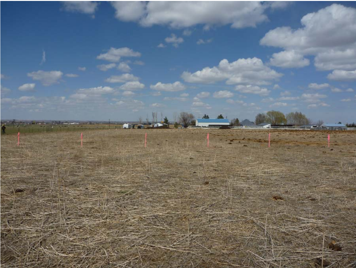
Pierson Tank Battery18-34 Location North NWNE Section 34-4N-66W 04/09/10
