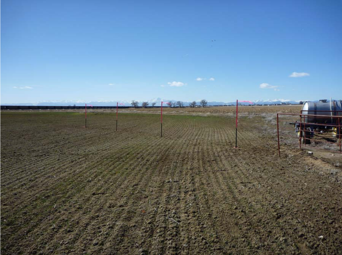
Spaur Tank Battery 41-7 Location West SENE Section 7-4N-67W 03/12/10
