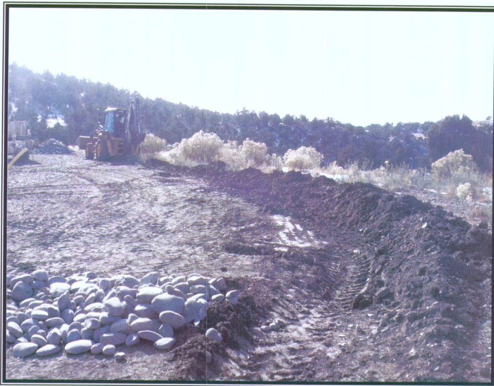
Photo 1: Construction of the ditch channel.
