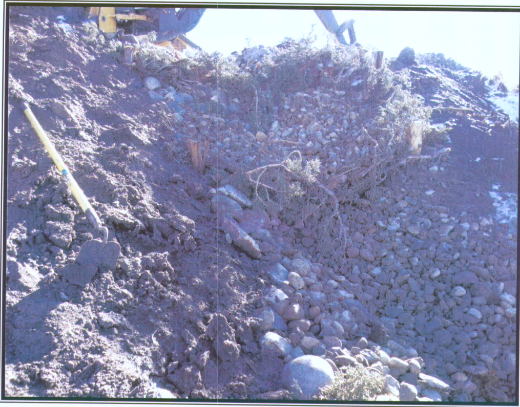
Photo 5: Gravel being placed on rock rundown.
