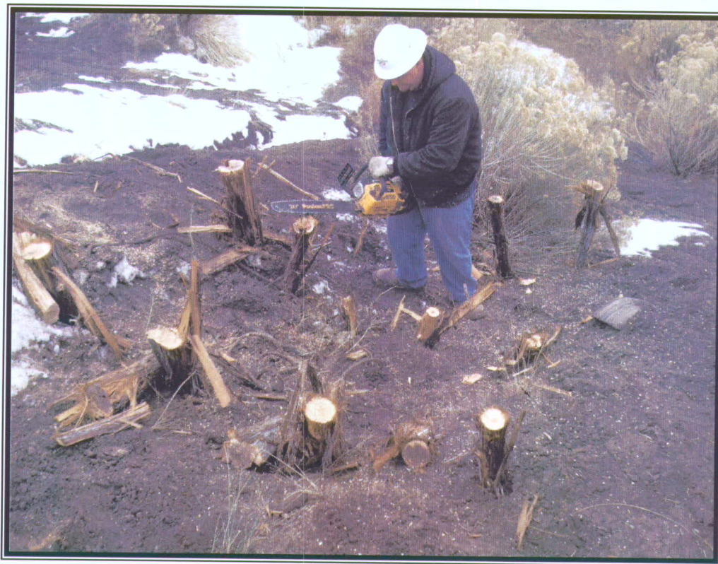
Photo 3: Trimming the pickets in the rundown.
