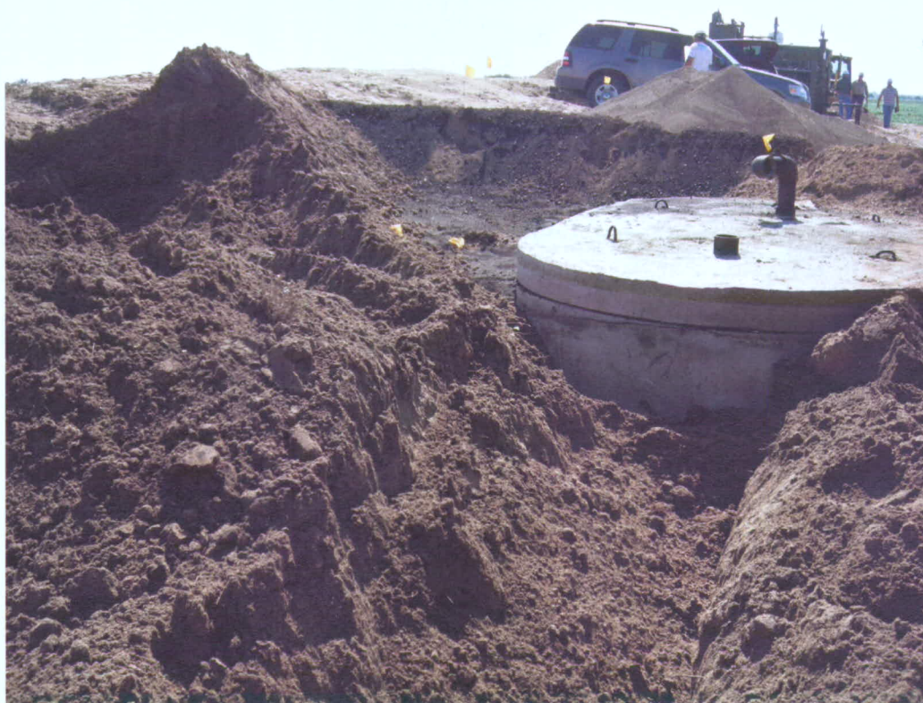
Photograph 2: Excavation of impacted soils adjacent to the water vault.
