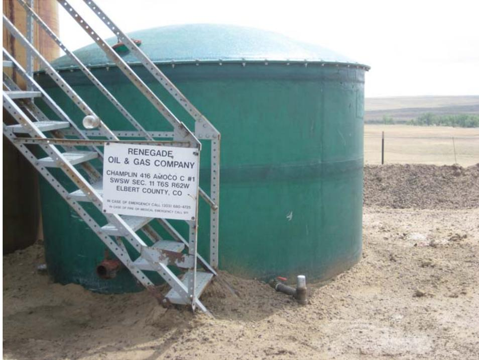
Photo 1. Covered fiberglass water tank
