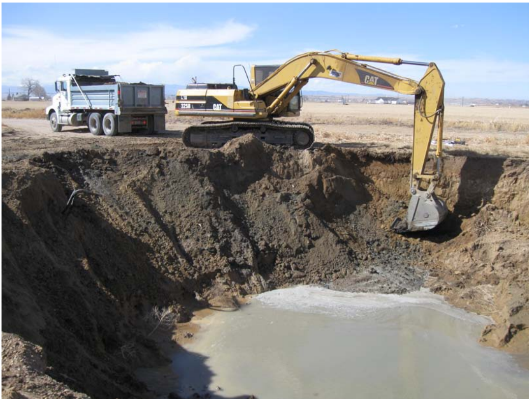
Photograph 2: Excavation of impacted soils on the west wall. View is west.
