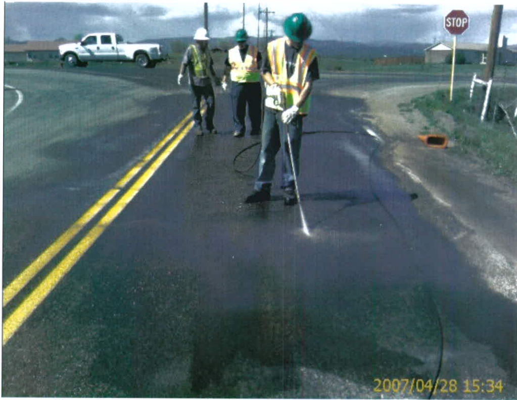
Photo 3: Pressure washing intersection of CR 307 and Hwy 172
