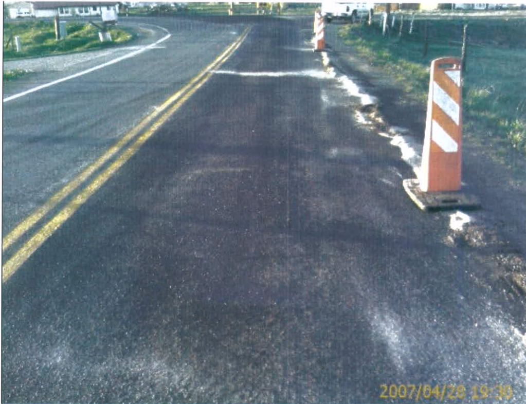
Photo 5: Oil absorbent crystals placed at intersection of CR 407 and Hwy 172
