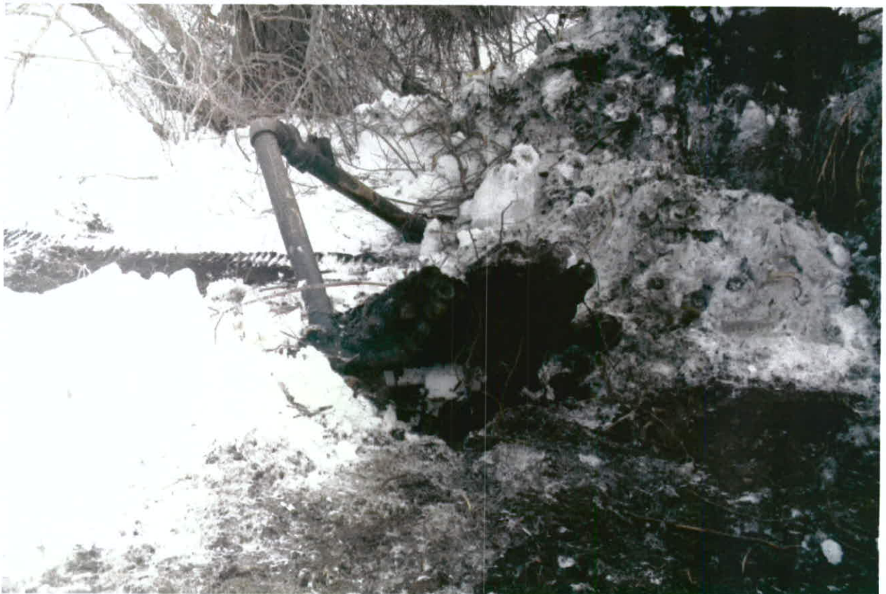
Photo 6 – View looking north at load out piping as it is removed.
