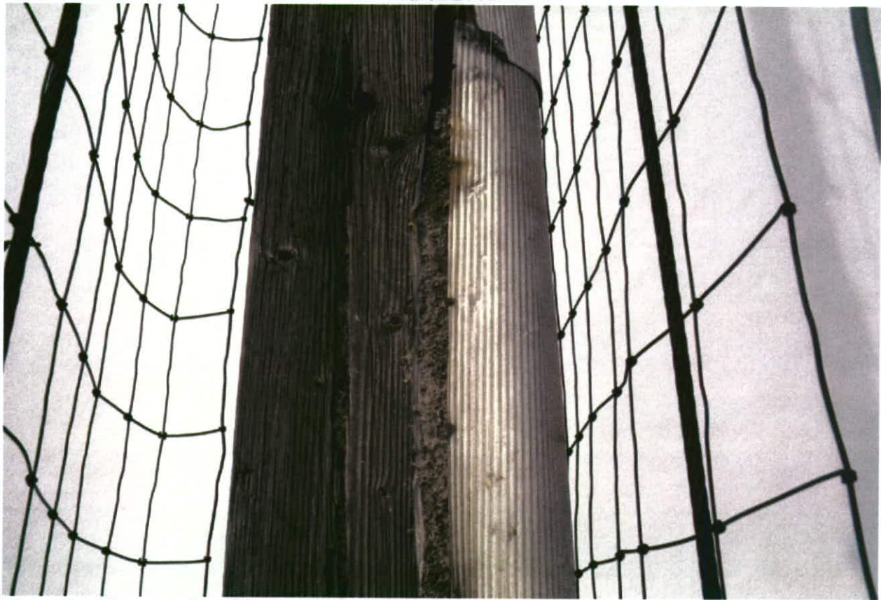
Photo 5 – Close up view of opened seam in metal jacket around asbestos insulation
