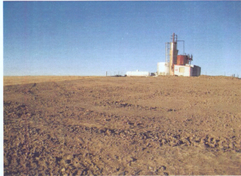
Photo # 27 – Evaporation pit area after backfilling
