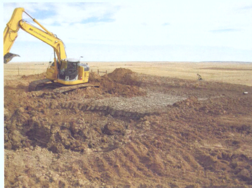
Photo # 24 – Excavation of evaporation pit bottom materials
