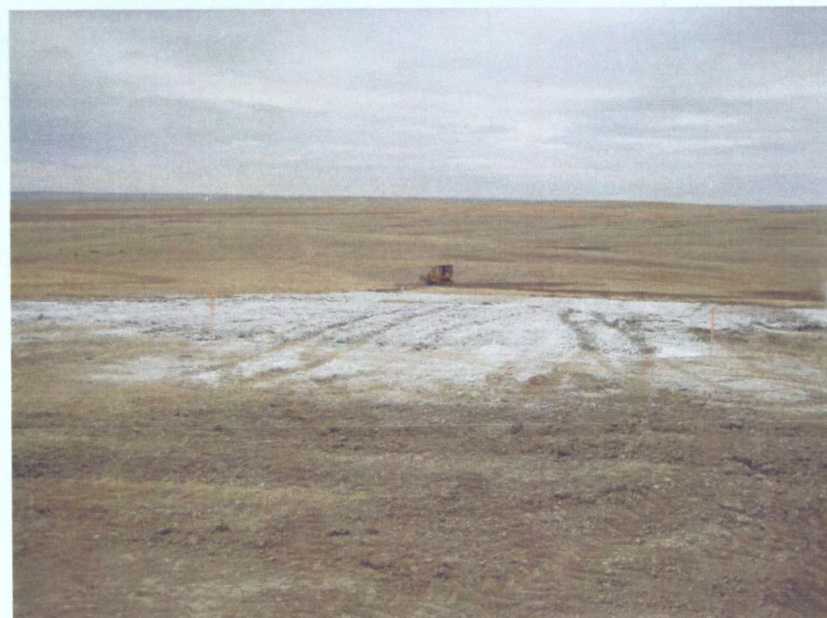
Photo # 30 – Application of gypsum and ripping
