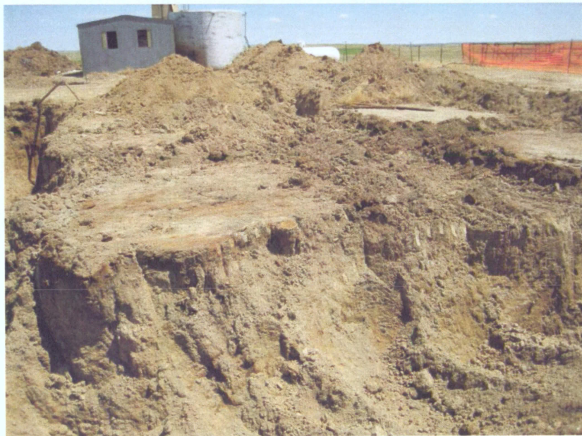
Photo # 14 – Tank berm area excavation
