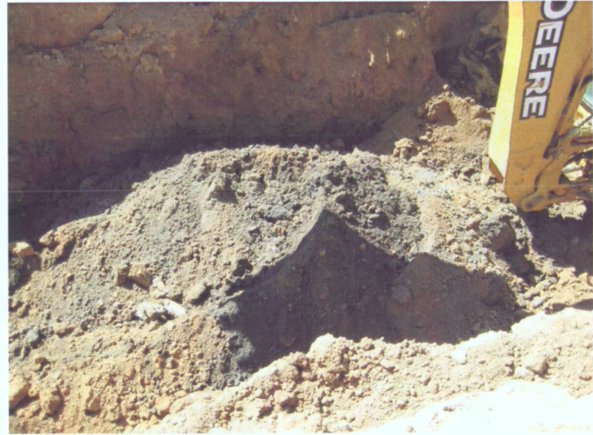
Photo # 11 – Petroleum-Impacted soils in tank berm area
