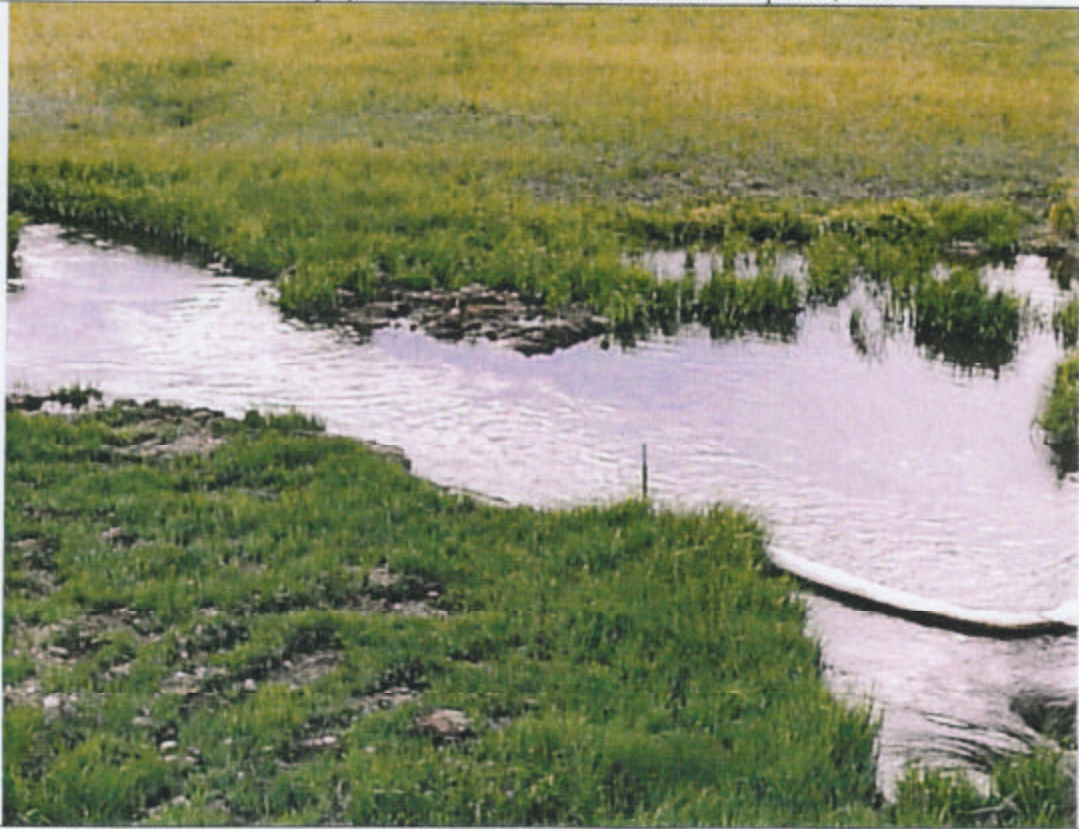
Photo 8 – Absorbent booms placed at Hell Creek Underflow Dam #1 – April 25, 2006
