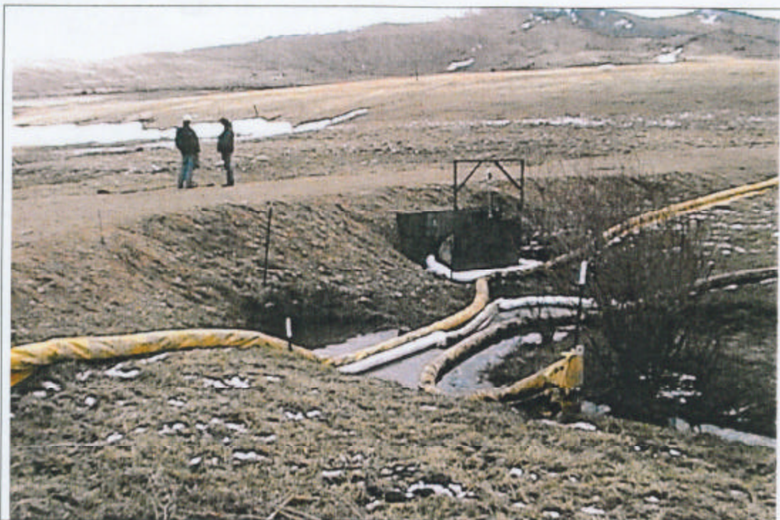
Photo 3 – Absorbent booms deployed at Hell Creek Underflow Dam #1 – April 25, 2006
