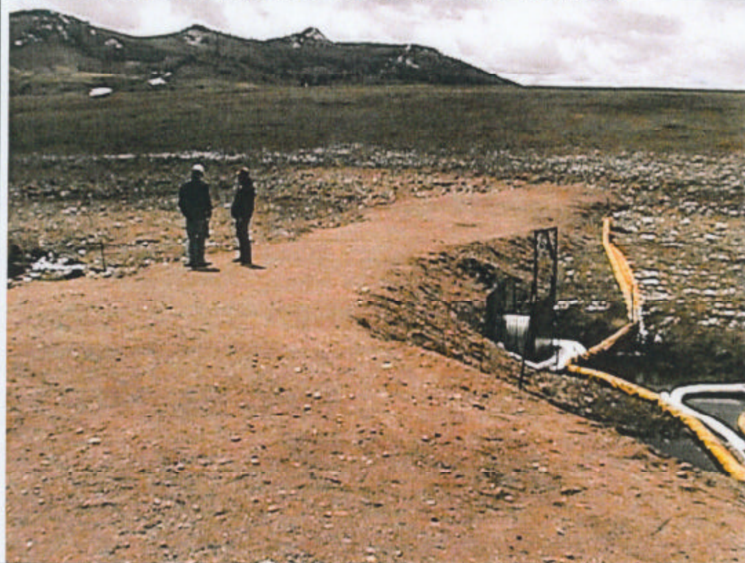
Photo 4 – Absorbent booms placed at Hell Creek Underflow Dam #1 – April 25, 2006
